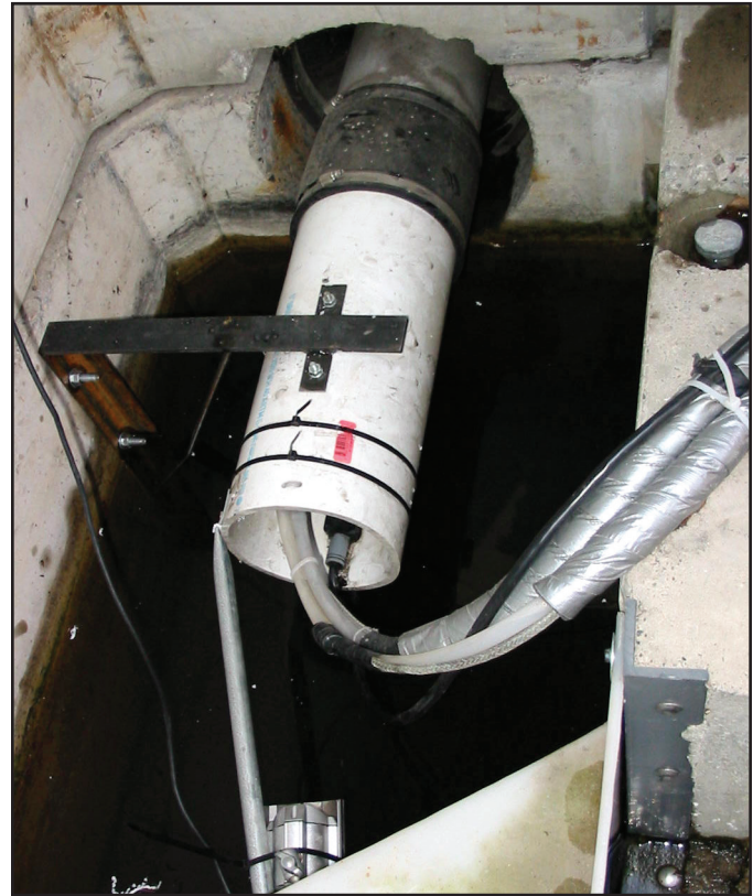
Figure 6. Inlet pipe with stabilization bar.
