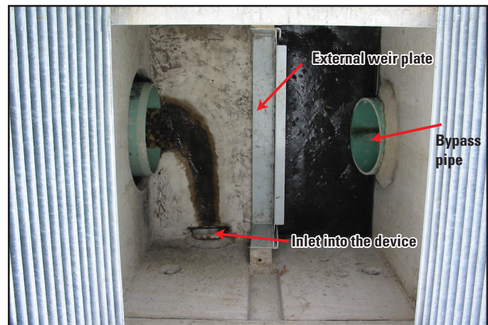
Figure 2. Flow-splitter box upstream from the stormwater-filtration device, representing the inlet pipe, the overflow weir, and the bypass pipe (top view).
