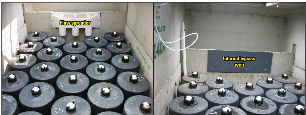
Figure 4. The flow spreader and the modification made to the internal bypass weir of the stormwater-filtration device. Each black cylinder contains a filter cartridge.
